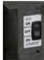
Water heater power switch
