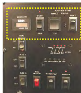
Command Center Panel
